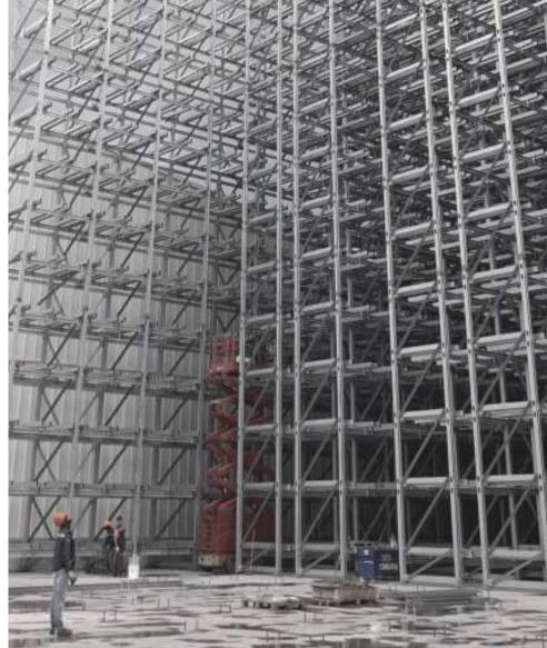
\*Structural assembly for automated warehouses
